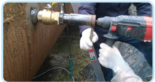
Insertion Transducer Installation
